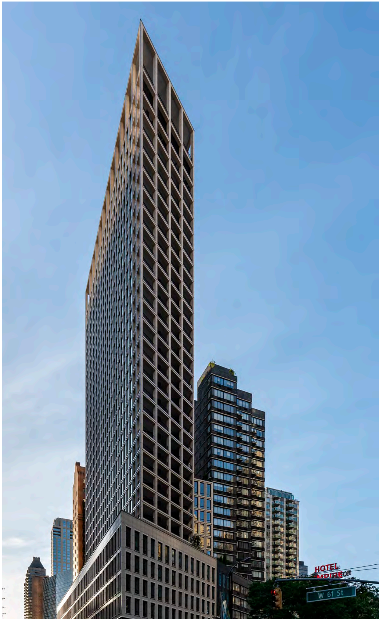
Foto: Field Condition for Shildan Group | SOM Architects | Broadway 1865, New York
